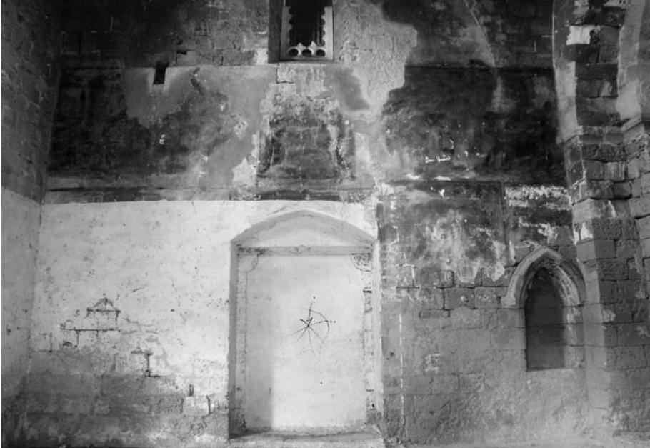
Fig. 10: Interior of the Armenian church, Famagusta. View of the north wall with whitewashed lower areas. Note the gothic piscina to the right (Photo Wilbert “Skip” Norman)
