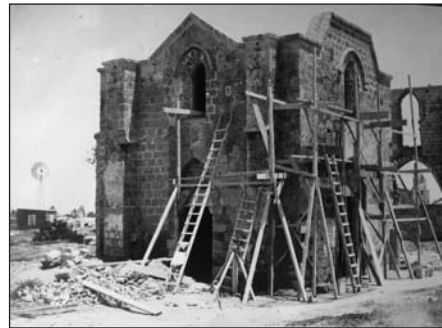
Fig. 6: Photograph by T. Mogabgab during 1930s restoration work (the Mogabgab Archive, Famagusta)
