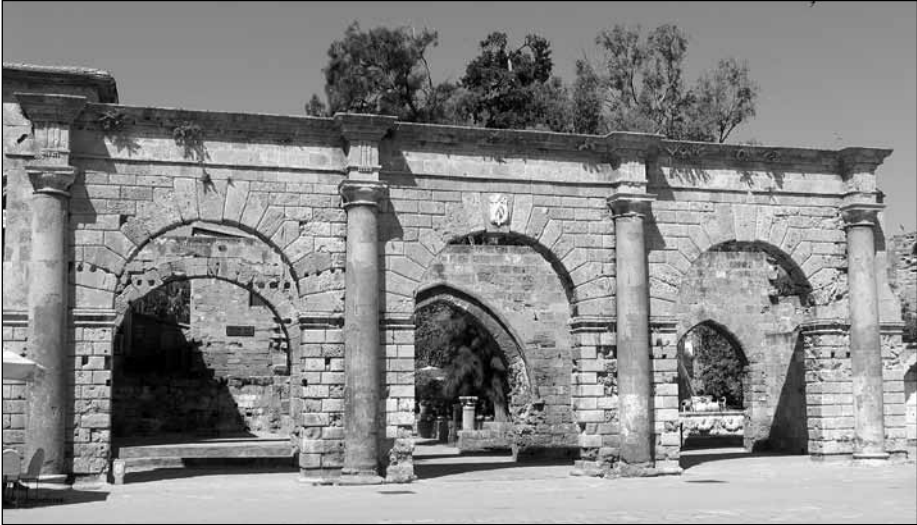
Figure 1. The Triple-arched Gateway of the Palazzo del Proveditore , Famagusta, with Four Granite Spolia Columns from the Greco-Roman City of Salamis – Langdale
