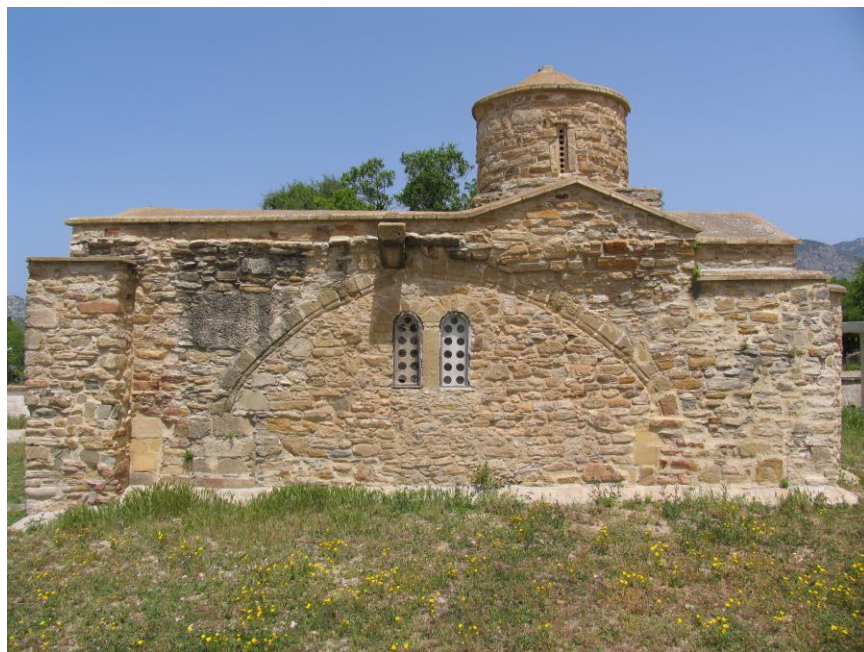
Fig. 15: Profile of early arch in the south side of the church of the Panagia in Kampyli/Hisarköy, Cyprus
