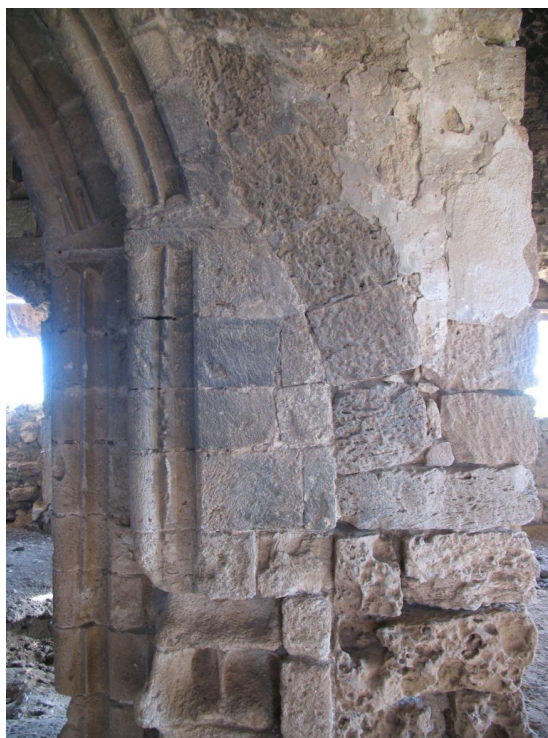
Fig. 5: Piers of the 14 th century dome, showing seam between the original masonry and masonry added in the 16 th century
