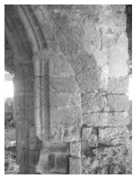
Fig. 5: Piers of the 14th century dome, showing seam between the original masonry and masonry added in the 16th century
